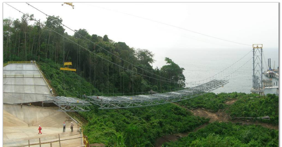
suspender cables and deck sections erected by 40T 'Hiline'
