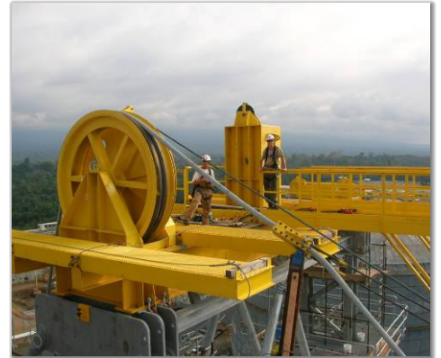
8ft dia. roller assembly for installing the main cables
