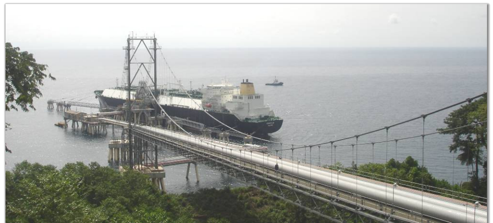
first LNG shipment June 2007, six months ahead of schedule. this tanker loaded 140 mil. cu. m in 14 hours
