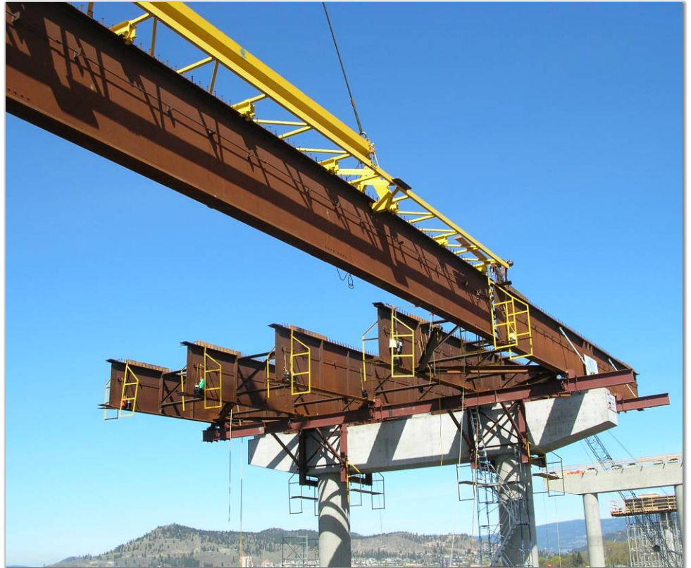
specialized support brackets stabilize girders at piers until the closure girders are erected
