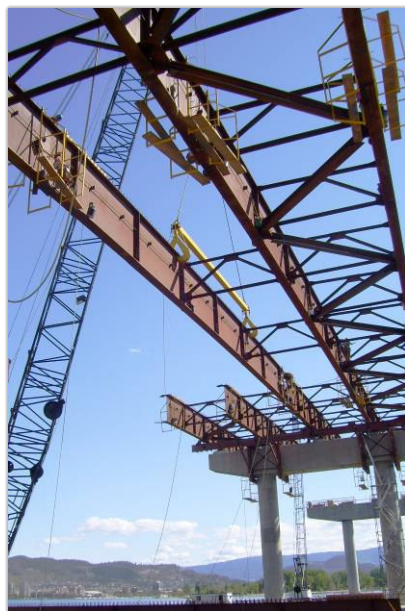
specialized support brackets stabilize girders at piers until the closure girders are erected
