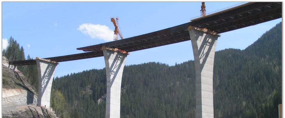
the launch system at the west abutment
