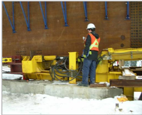
the launch system at the west abutment
