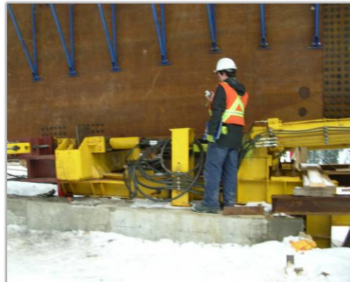
the launch system at the west abutment
