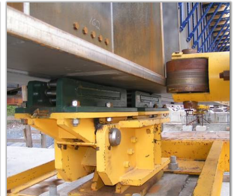
roller brackets and guide system at piers
