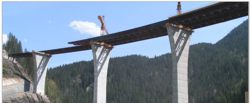
the launch system at the west abutment
