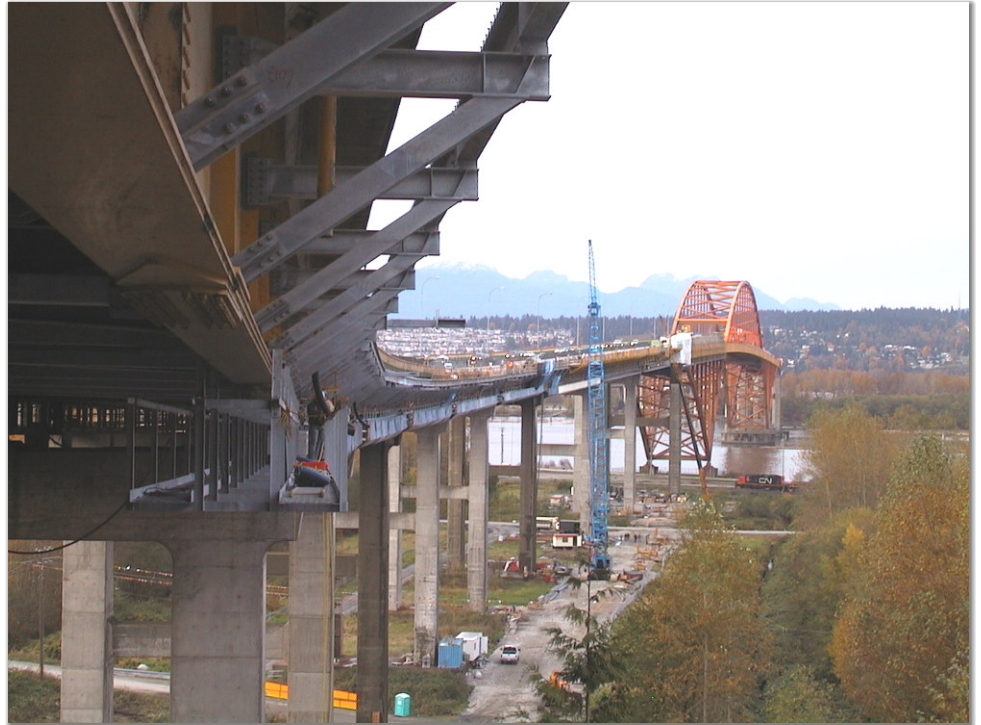
cantilevered brackets to accommodate extra HOV lane
