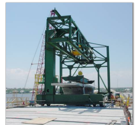
The "Florida Lifter" picking up to 85 ton pre-cast segments and setting them on rollers on under-slung assembly girders
