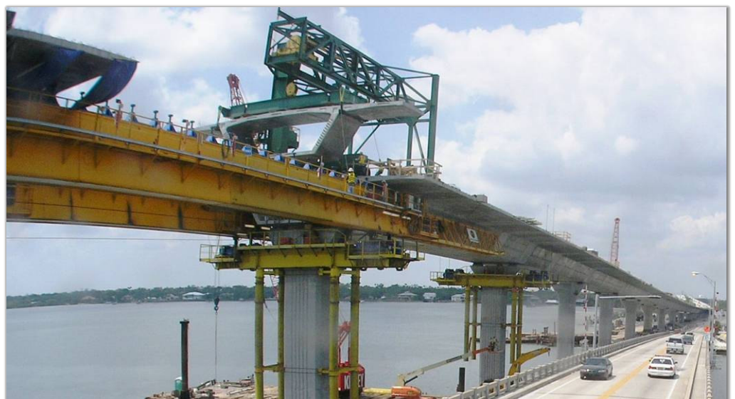
The "Florida Lifter" picking up to 85 ton pre-cast segments and setting them on rollers on under-slung assembly girders
