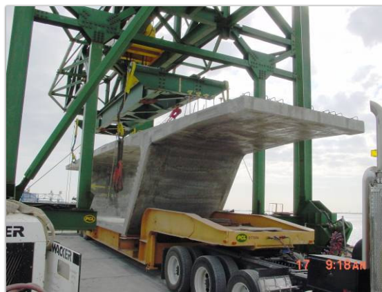
The "Florida Lifter" picking up to 85 ton pre-cast segments and setting them on rollers on under-slung assembly girders
