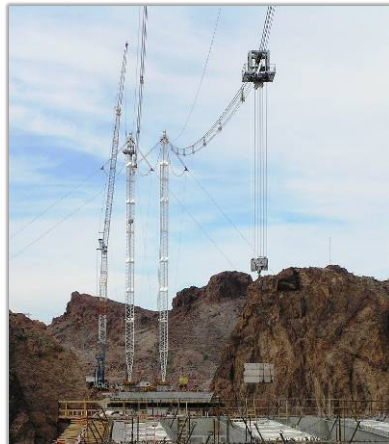
First test lift
