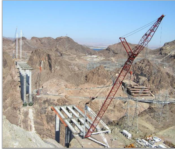
S-70 stiff-leg derrick adapted with a Manitowoc boom
