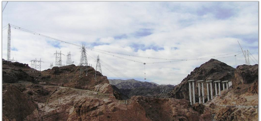
Twin 50T luffing cableways servicing a 2500' span
