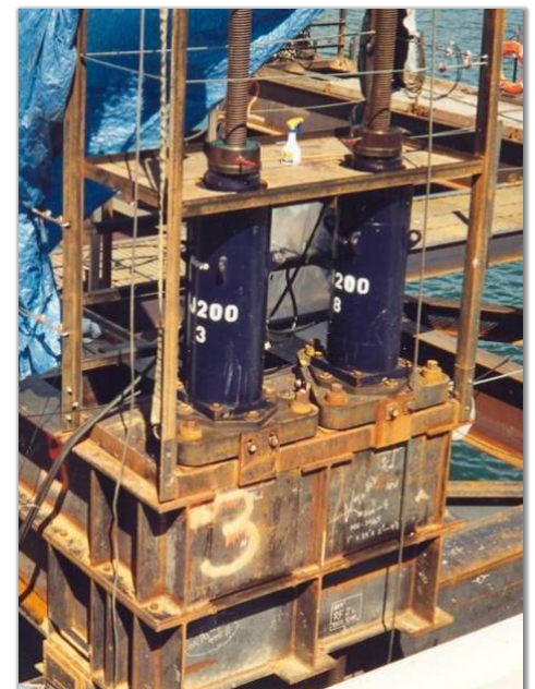
Structure lowered by jacks and threaded rods
