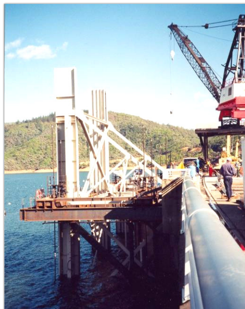
Shoring hung from dam supports erection
