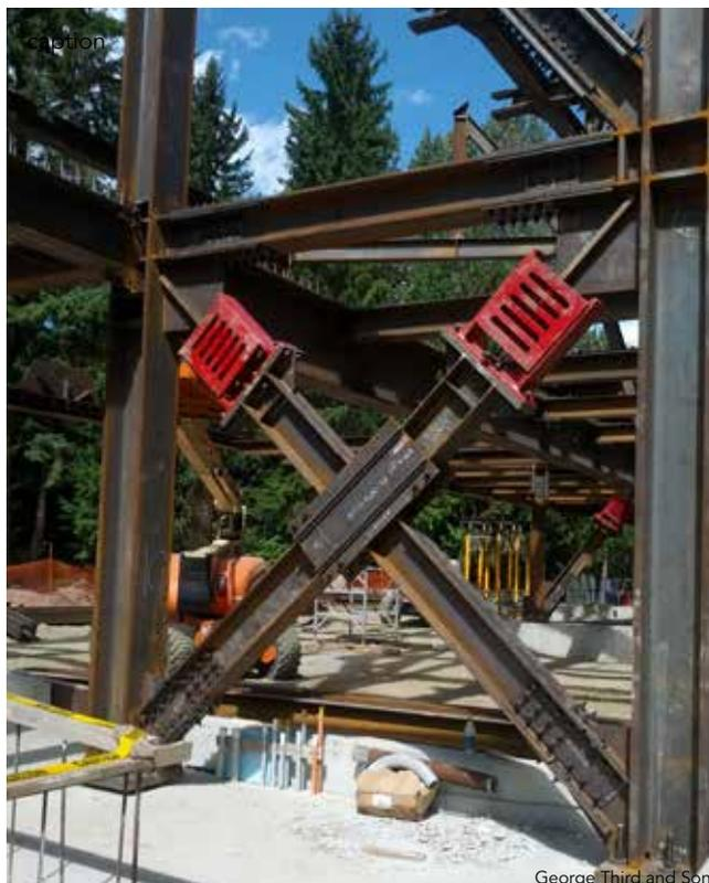
► The various components of the SYC. The moniker comes from the original prototype's resemblance to a scorpion, with the connectors forming the "claws."
